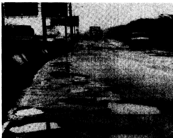
Photo credit: American Society of Civil Engineers
