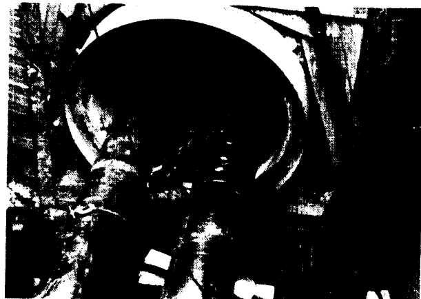
e) High-temperature district heating pipe during construction
