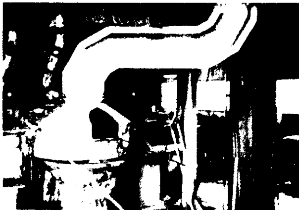
This hood in a secondary lead smelter illustrates the use of local exhaust ventilation
